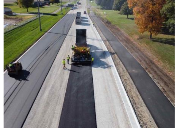
Aerial view of first layer of asphalt being laid in County Hwy II (10/19/2021)
