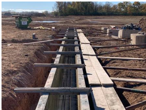
Foundation wall forms (10/25/2021)
