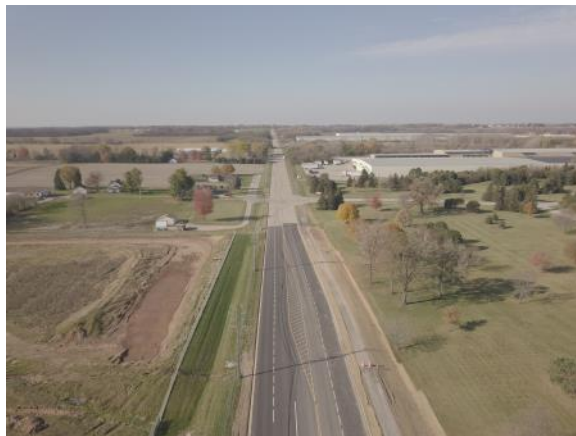
Completed County Hwy II paving West of school entrance (10/27/2021)
