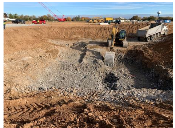
Orchestra pit excavation (10/25/2021)
