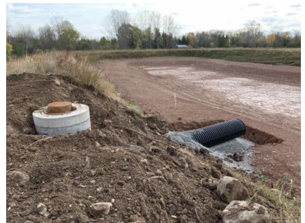
Emergency overflow outlet in retention pond (10/19/2021)
