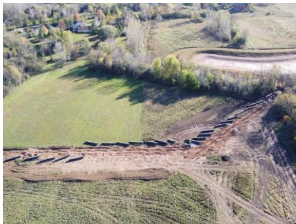
Storm piping exiting from retention pond to wetlands (10/19/2021)
