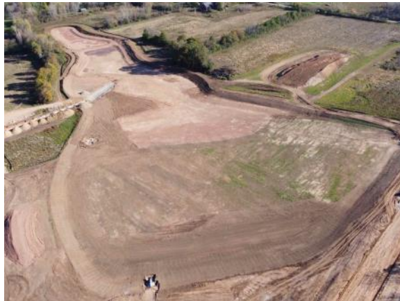
Aerial view of entire retention pond (10/19/2021)
