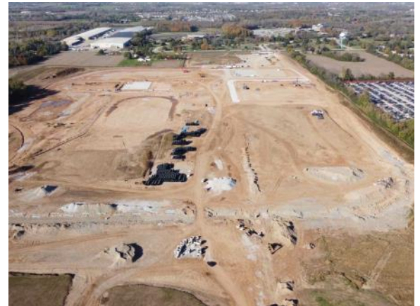
Aerial view of site looking North (10/19/2021)
