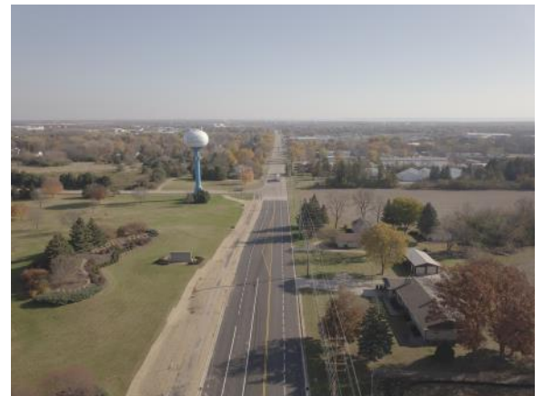
Completed County Hwy II paving East of school entrance (10/27/2021)
