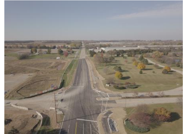
Completed County Hwy II paving at Rocket Way intersection (10/27/2021)
