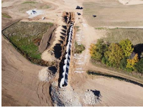
Storm water flume leading into the retention pond (10/19/2021)
