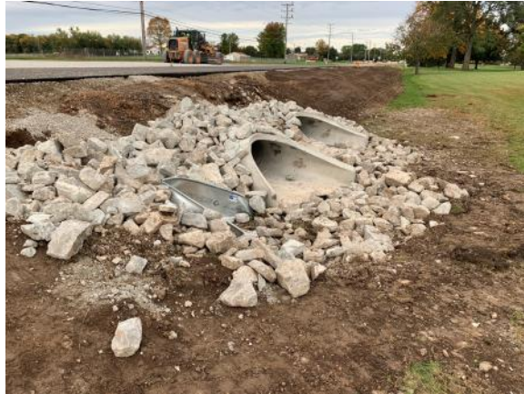
Concrete endwall installation next to County Hwy II (10/25/2021)
