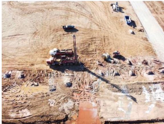
Drilling for geothermal field (10/19/2021)
